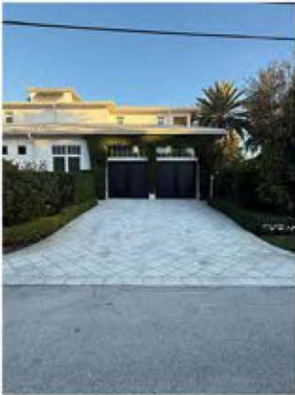
Garages with steep entry
