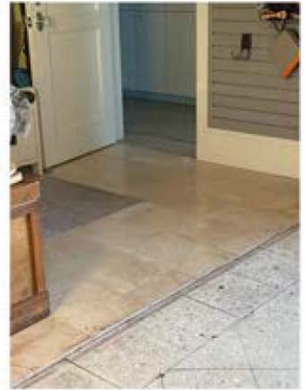
Close-up of accessible entry
