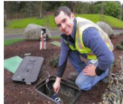
New Meter Installation
