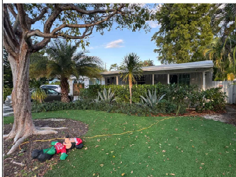
WEST: ANGLED FRONT STREET VIEW (OPPOSITE CARPORT)
