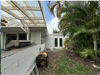
EAST: REAR OF HOUSE ABUTTING PROPERTY LINE
