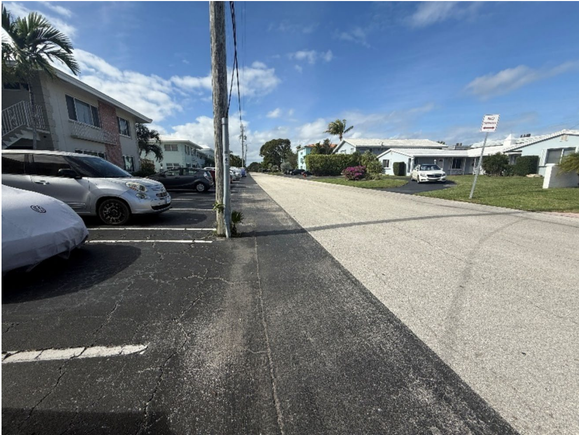
Photo 13 (12/17/25): Front of building, facing west, at Lexington Arms Co-op; 2830 NE 30 th Street. Photo is west facing. Existing parking, right-of-way/swale, and road conditions. This building is located on next property to the west of Lafayette Arms Co-op (project location).
