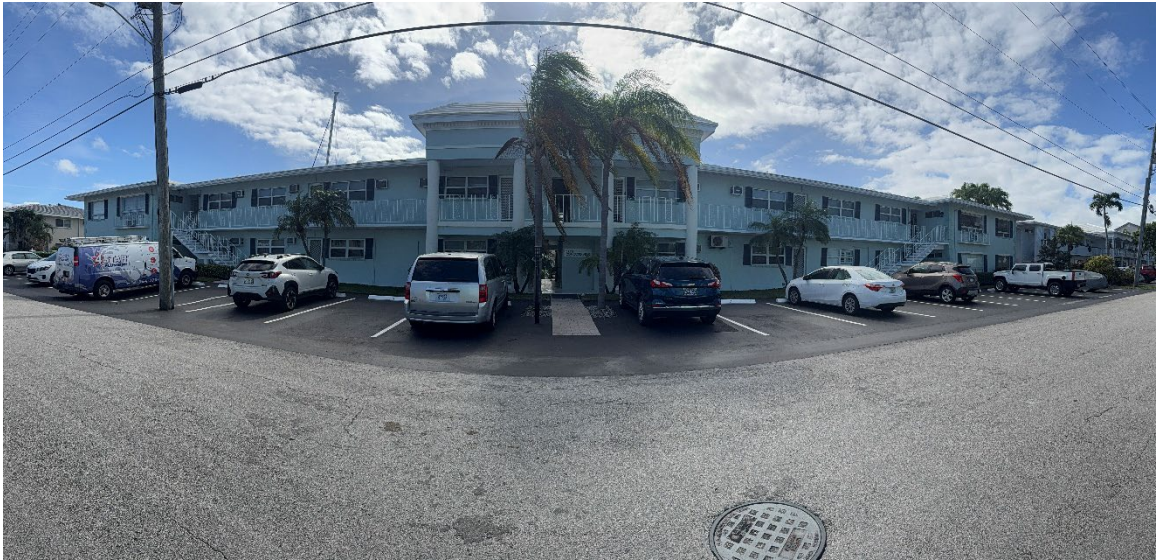
Photo 12 (12/17/25): Front of sister building, Concord Arms Co-op; 2830 NE 30 th Street. Photo is of north elevation. Existing parking and landscaping conditions. This building is located on two properties to the west of Lafayette Arms Co-op (project location).
