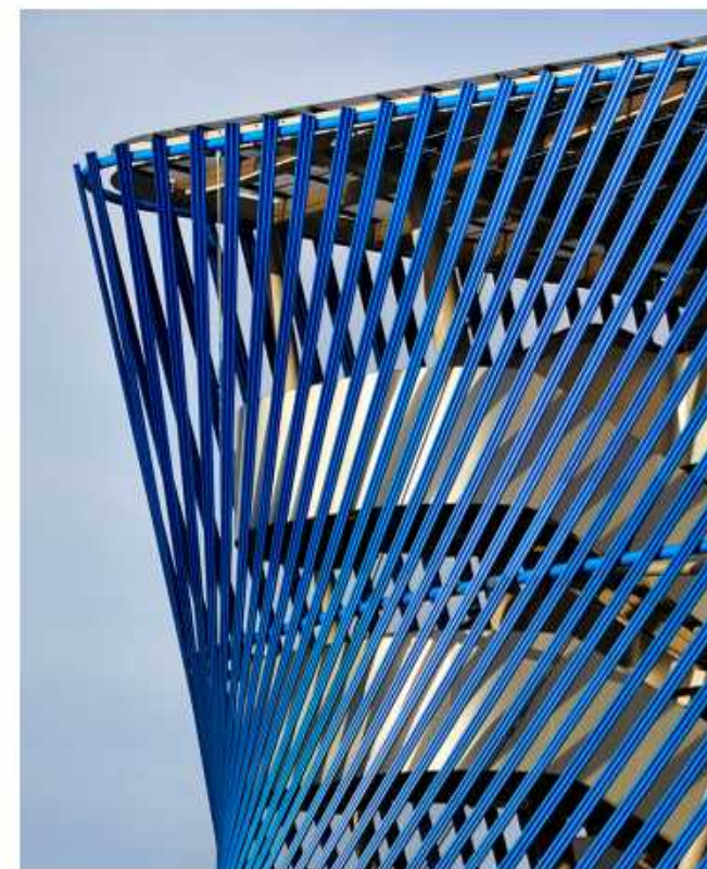
Brooks Scarpa Huber Architects, Angle Lake , 2017
