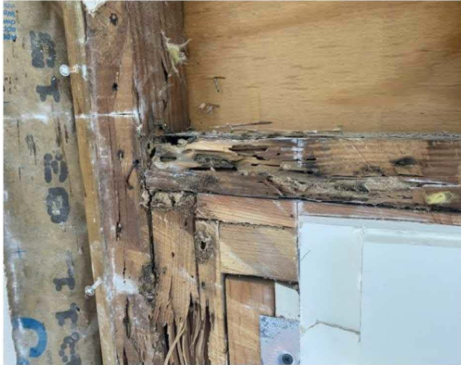
Photo 8: South Window Jamb at Header
