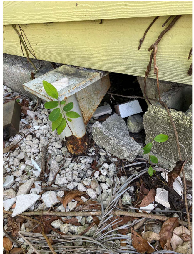
Photo 1: Pile at West Exterior Wall
