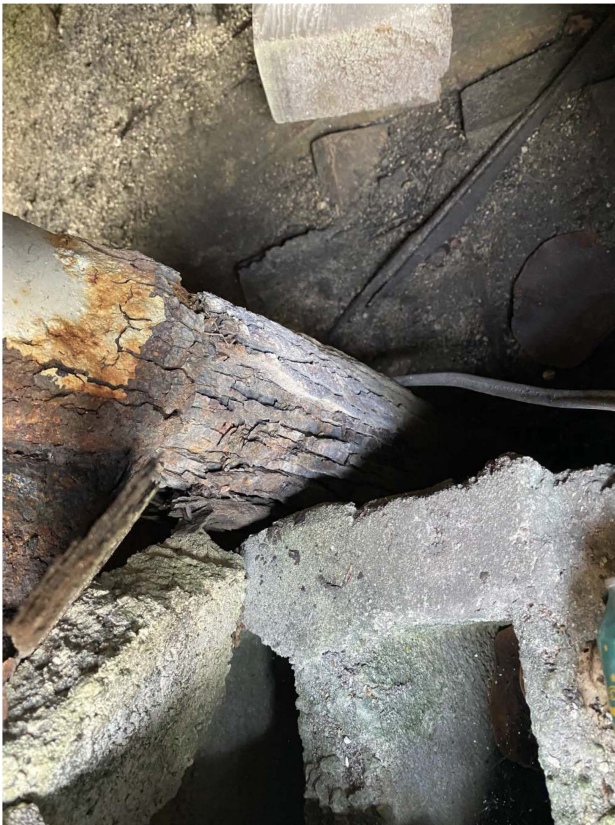
Photo 2: Pile at Southwest Corner
