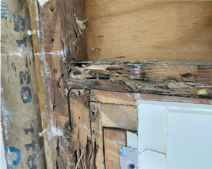
Photo 8: South Window Jamb at Header
