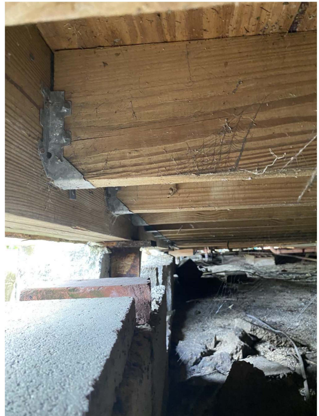
Photo 3: Floor Framing at West Exterior Wall
