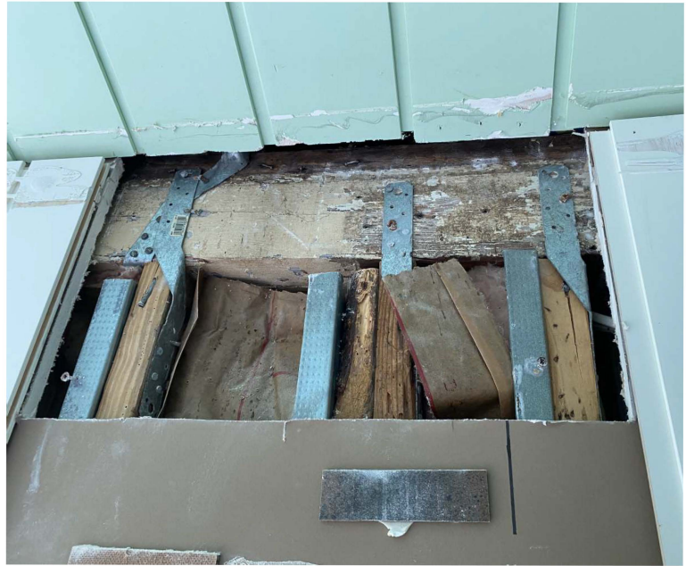
Photo 4: South Wall Framing at Bedroom
