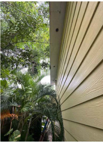
EXISTING WOOD SIDING - PHOTO 1.
