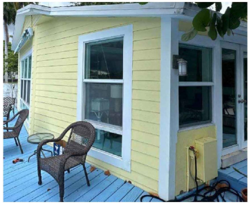
EXISTING WOOD SIDING - PHOTO 2
