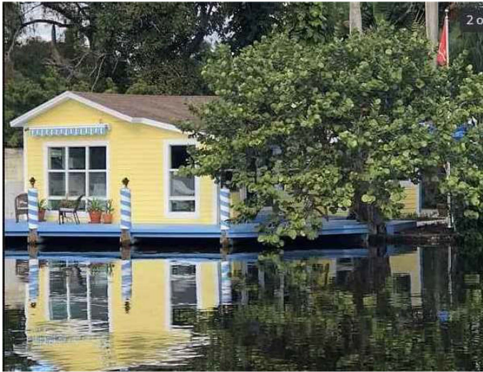
PHOTO #3: EXISTING SOUTH VIEW
