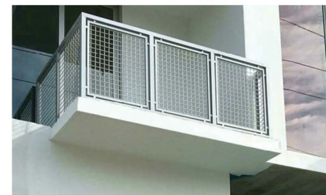
7- SQUARE STEEL MESH BALCONY
