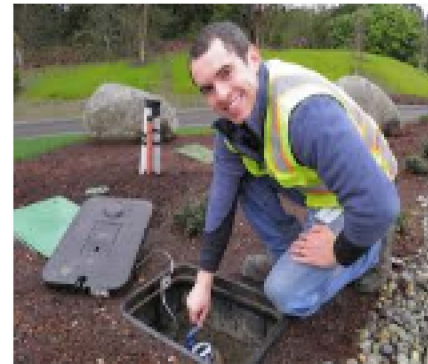
New Meter Installation
