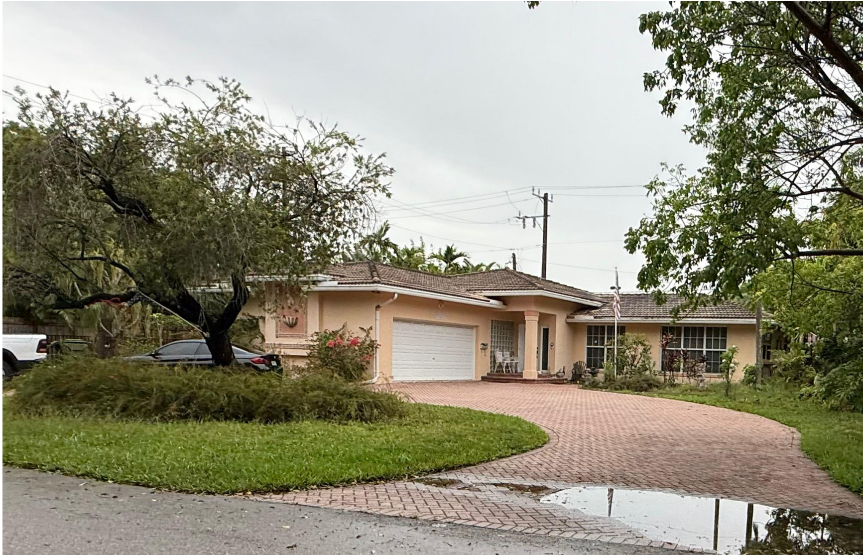
2537 NE 8th St, Fort Lauderdale, FL 33304 (Neighbor opposite corner lot, NW Street View)
