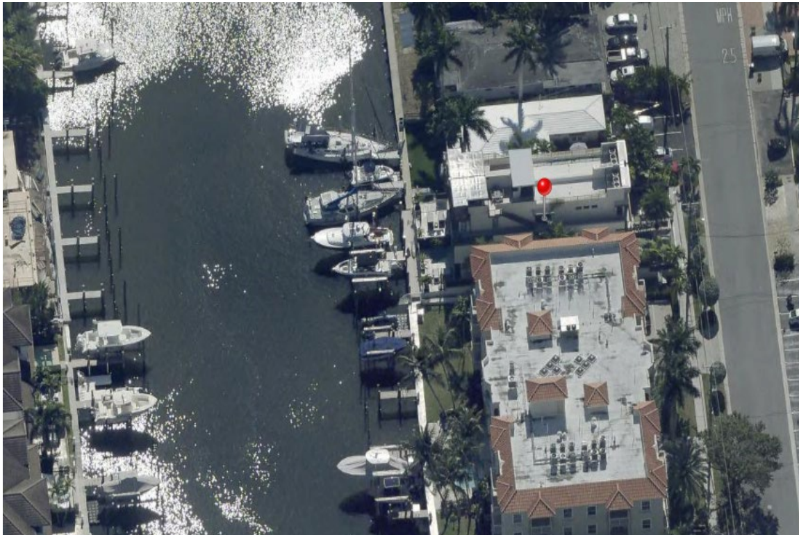
2. Northern portion of property, facing south.
