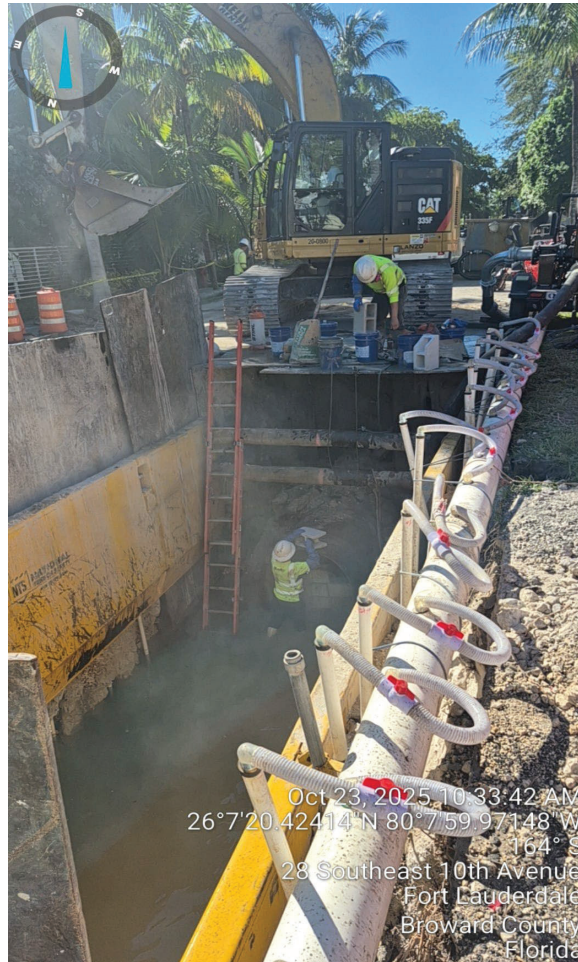
P12799 - Rehabilitation/Replacement of 48"/54" Force Main along SE 9 th and 10 th Avenue to GTL
