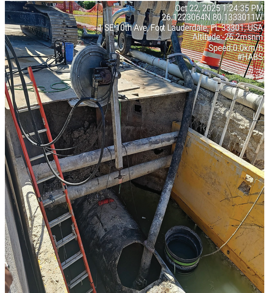
P12799 - Rehabilitation/Replacement of 48"/54" Force Main along SE 9 th and 10 th Avenue to GTL
