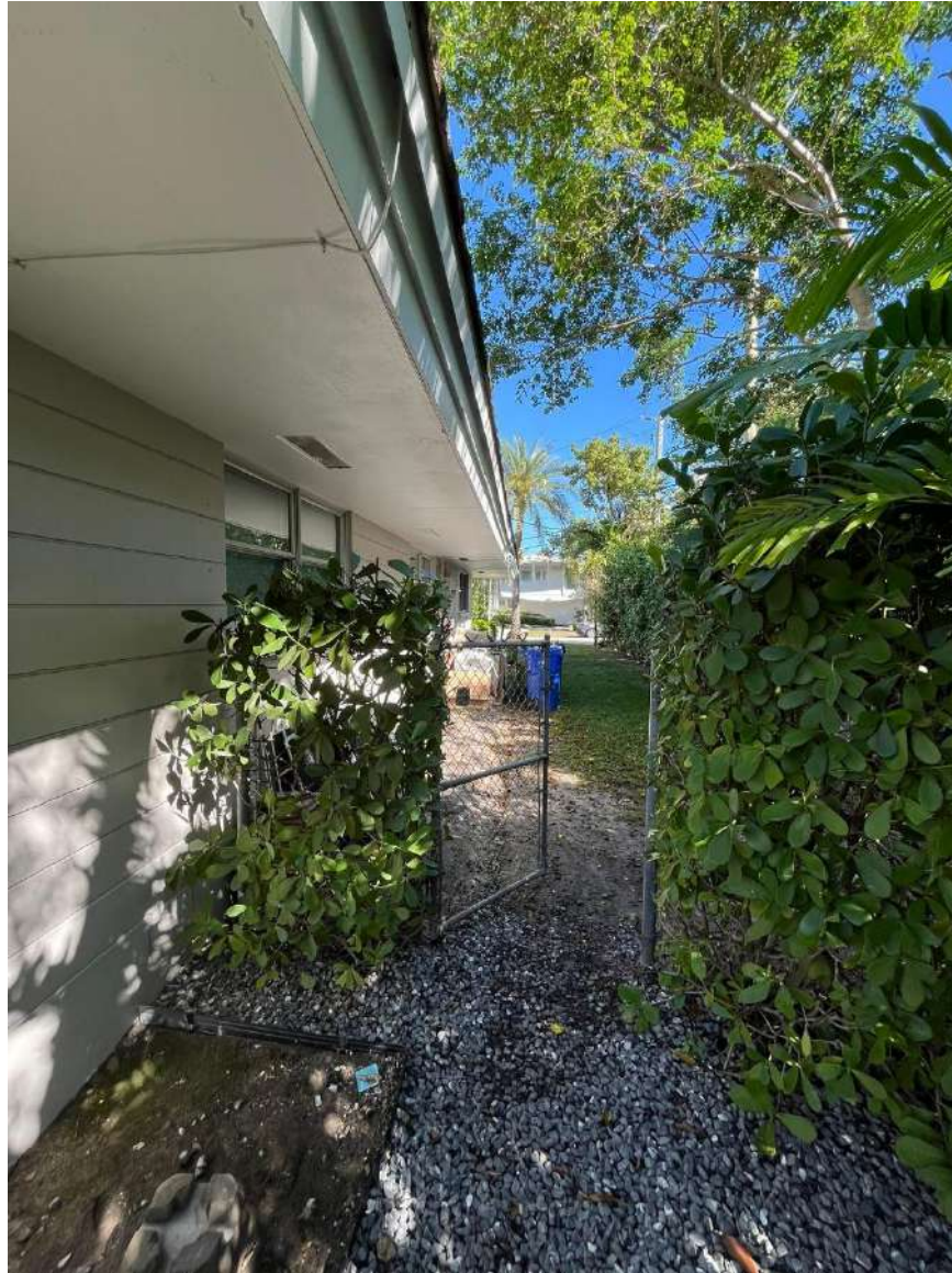
2600 NE 8th St, Fort Lauderdale, FL 33304 (Side View of Addition)
