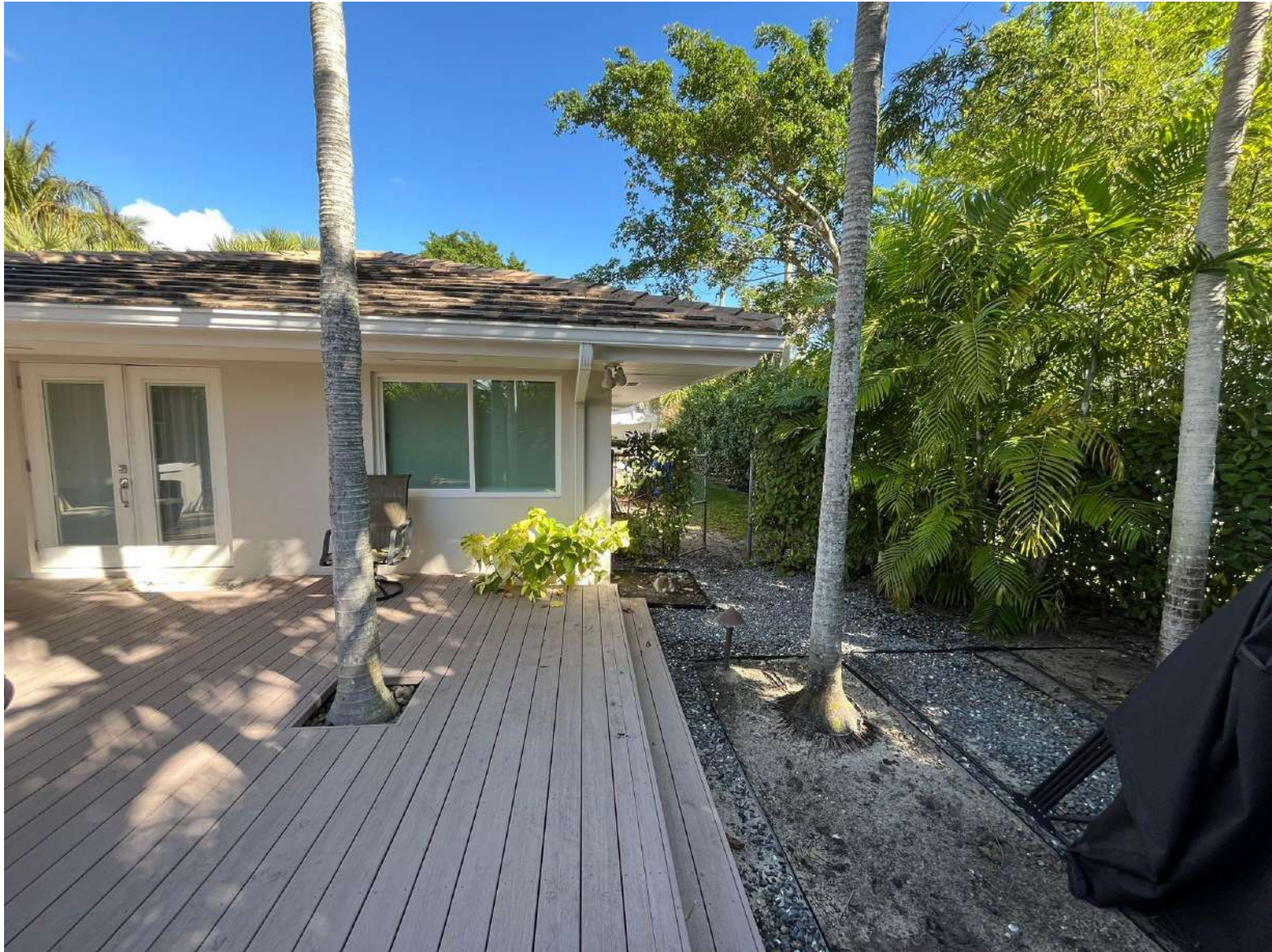
2600 NE 8th St, Fort Lauderdale, FL 33304 (Side View of Addition)
