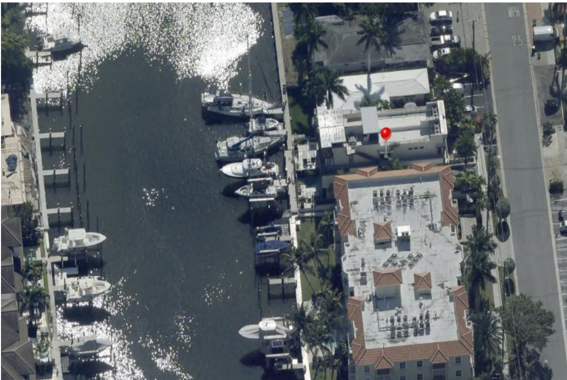
2. Northern portion of property, facing south.
