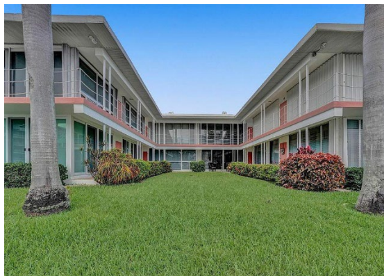
Photo from Interior Courtyard
