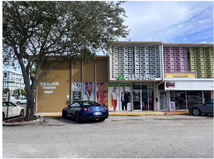
Photo: Current condition of the building.
