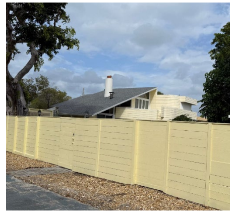
View looking northeast (rear)
