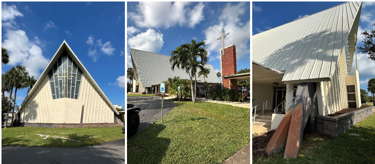
Photos of Existing Conditions
