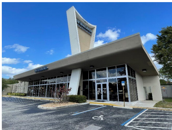
Photo of Existing Conditions
