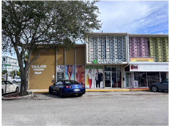
Photo: Current condition of the building. Source: Survey Team
