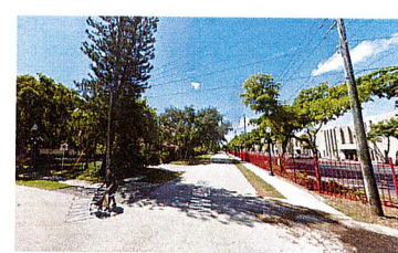
8 AR-01 AT NW CORNER OF SITE LOOKING SOUTH N.T.S.
