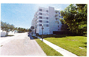
2 AR-01 AT SE CORNER OF SITE LOOKING SOUTH N.T.S.
