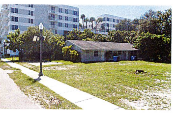
3 AR-01 AT SE CORNER OF SITE - EXIST. 1-STORY RESIDENTIAL BLDG. N.T.S.
