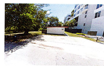
12 AR-01 AT SW CORNER OF SITE - EXIST. 2-STORY RESIDENTIAL BLDG. N.T.S.
