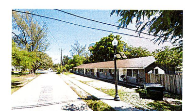
7 AR-01 AT NORTH SIDE OF SITE - EXIST. 1-STORY RESIDENTIAL BLDG. N.T.S.
