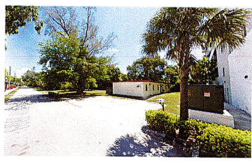
13 AR-01 AT SW CORNER OF SITE LOOKING NE N.T.S.
