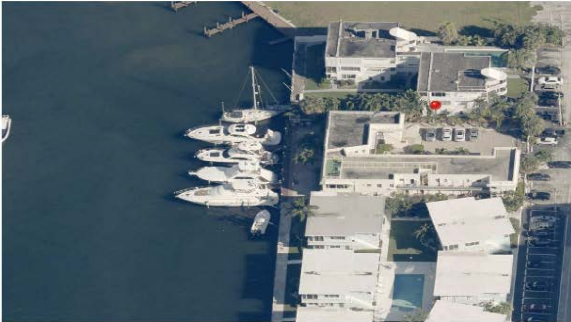
3. Eastern portion of the subject site, facing east along the New River Sound.
