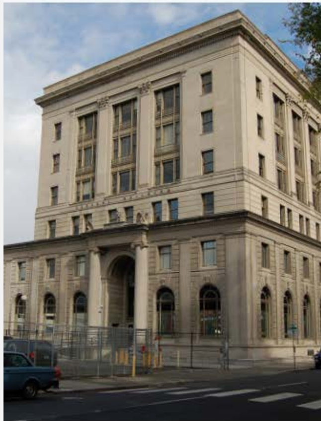
511 BROADWAY FEDERAL BUILDING PORTLAND, OR CONVEYANCE TYPE HISTORIC MONUMENT CONVEYED JANUARY 2014 CONVEYED TO CITY OF PORTLAND
