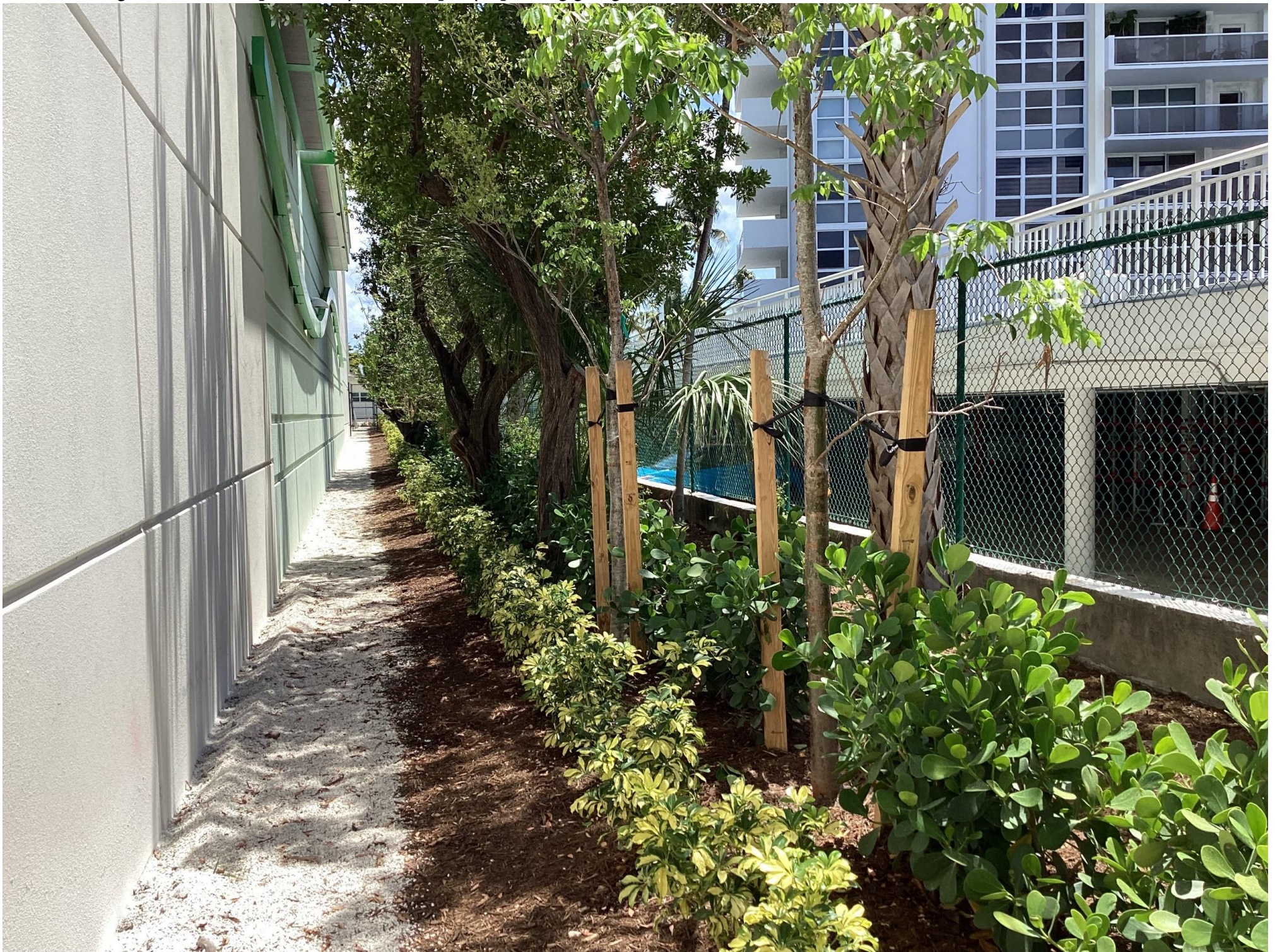
View looking east of landscape and Adjacent Property's parking garage wall
