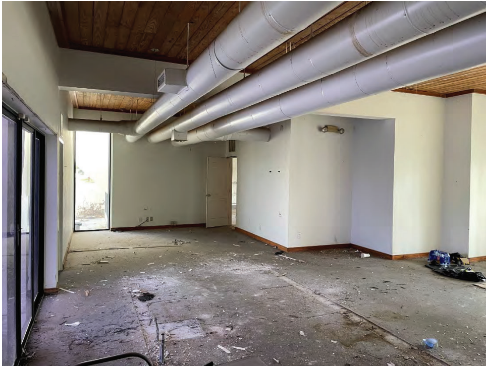
TYPICAL INTERIOR VIEW
