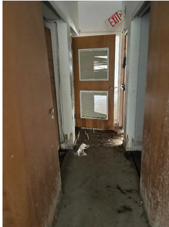
TYPICAL INTERIOR VIEW
