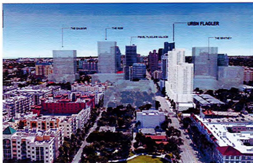
CONTEXT VIEW SOUTH
