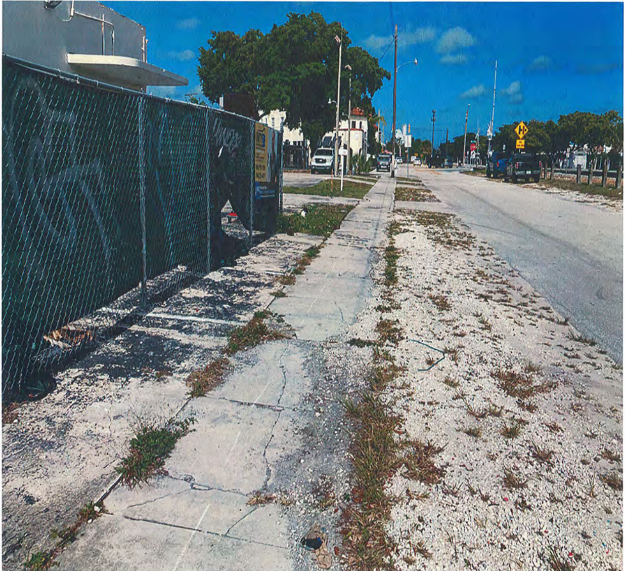
Existing Street Conditions at Proposed Site for "Progresso Park" Project
