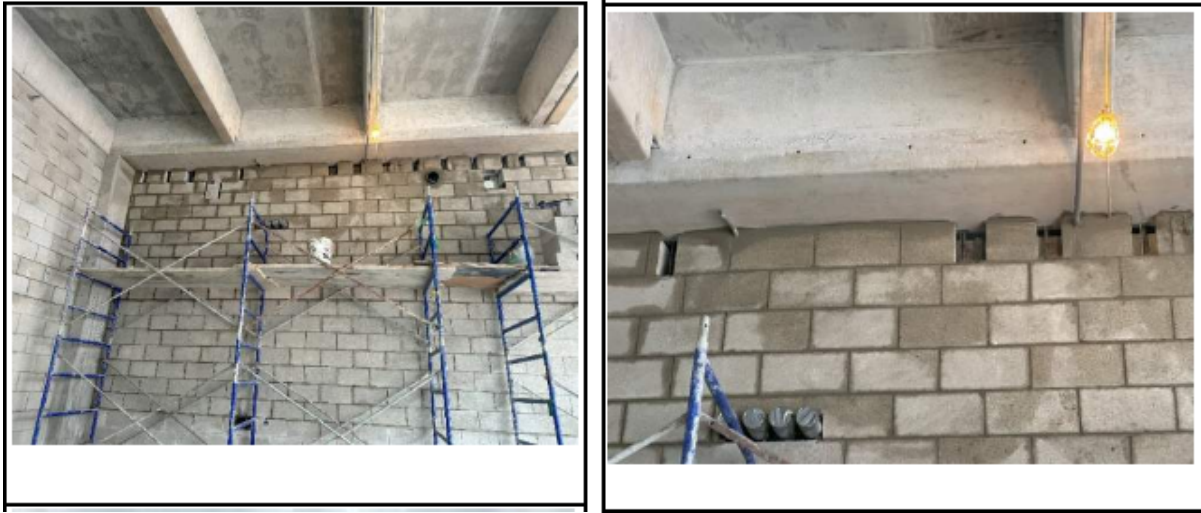
Figure 29. Photographs from Threshold Inspection Report No. 133 showing CMU wall at Level 1, Area D
