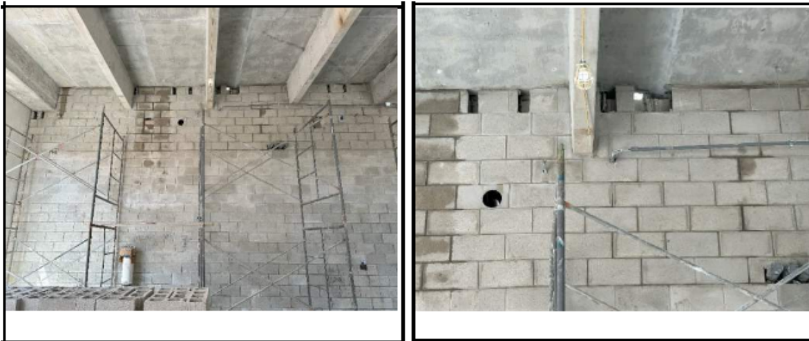
Figure 28. Photographs from Threshold Inspection Report No. 131 showing a wall that is nearly complete
