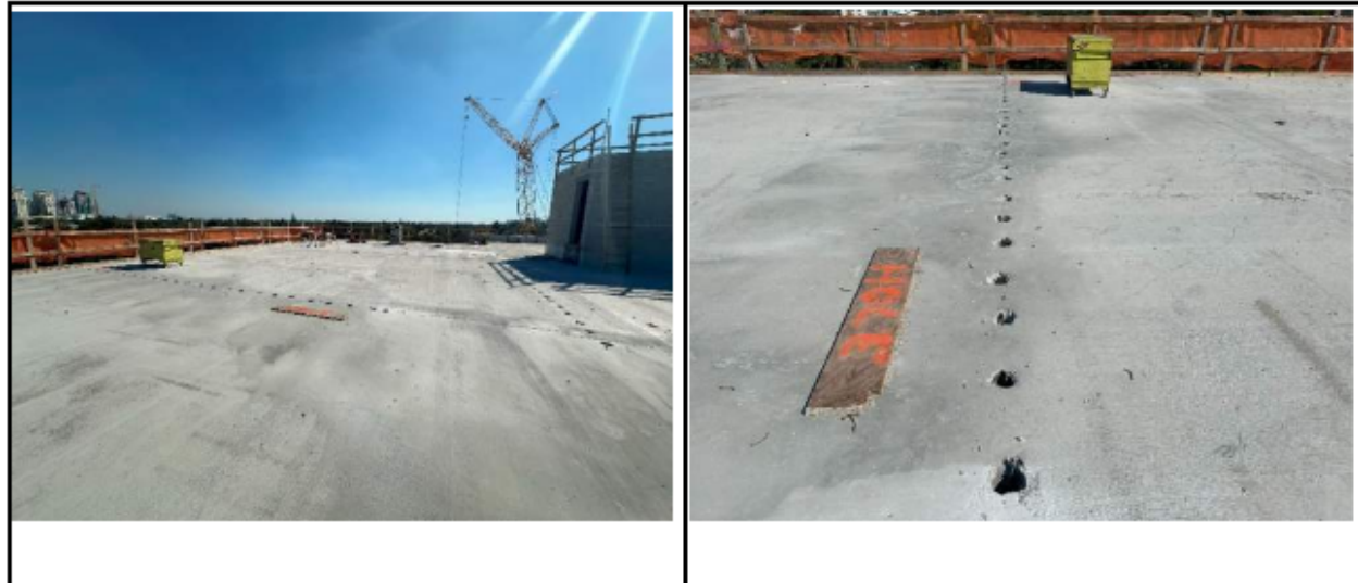
Figure 21. Photographs from Threshold Inspection Report No. 101. While not clearly stated in the report, these images are believed to be of the third floor slab
