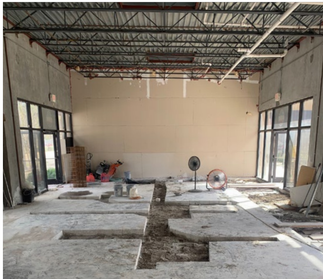
Jamaican Jerk Shack Construction
