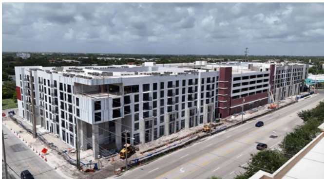
The Adderley mixed-use development Construction
