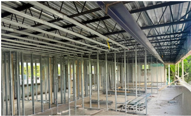
Construction of Mixed-Use Space at 1227 Sistrunk Blvd
