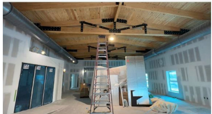
Construction of the Boys & Girls Clubs Teen Center
