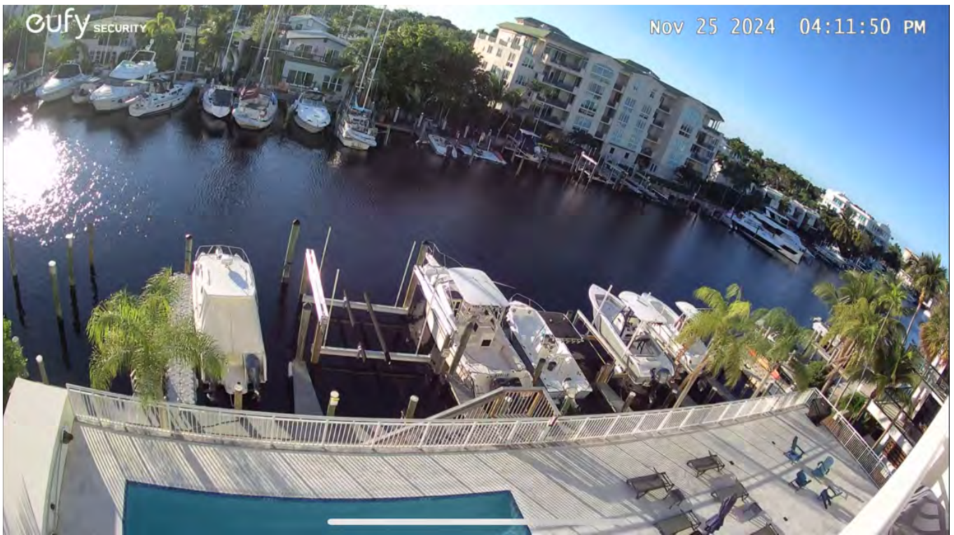
Aerial View of boatlift as currently installed
