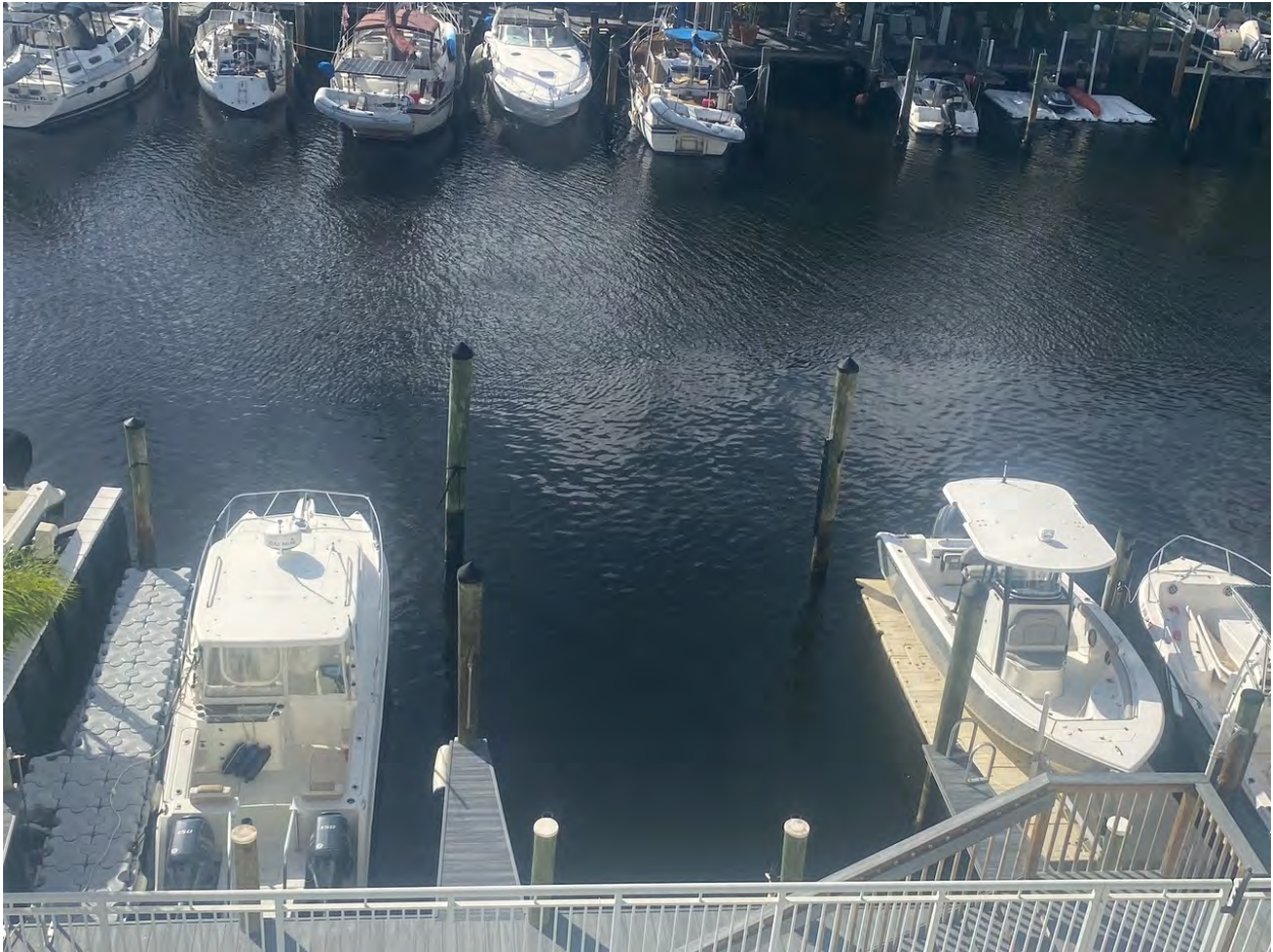
Project Site showing the existing mooring pilings
