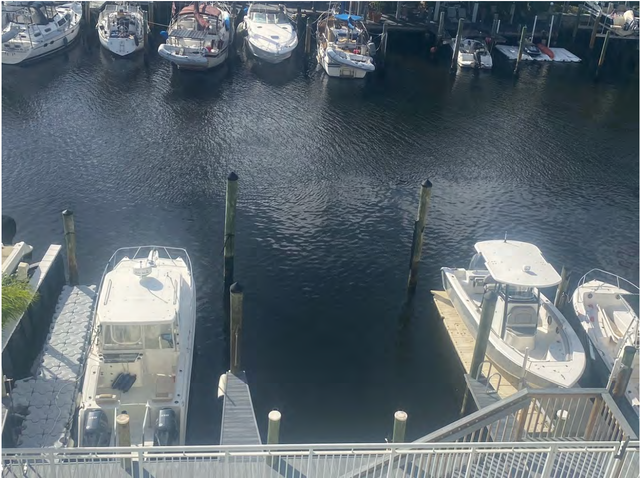
Project Site showing the existing mooring pilings
