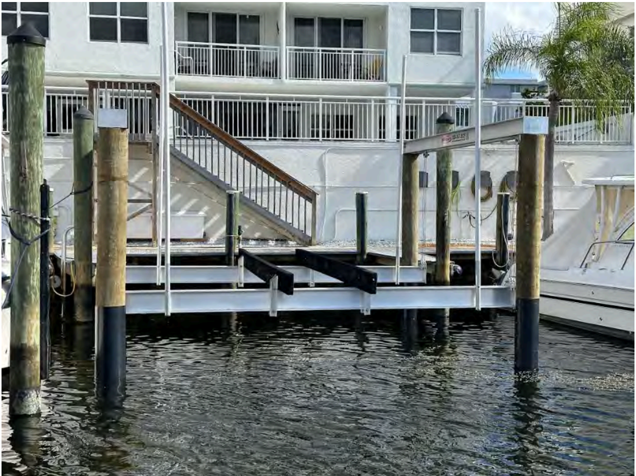
Boat Lift front view from canal
