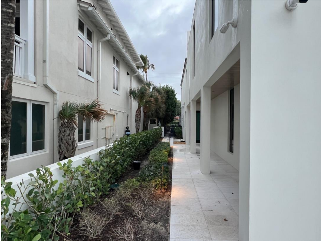
PHOTO 5: INTERIOR (SOUTH) SIDE; WEST VIEW
