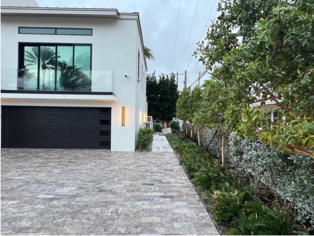
PHOTO 3: INTERIOR SIDE; SOUTH VIEW
