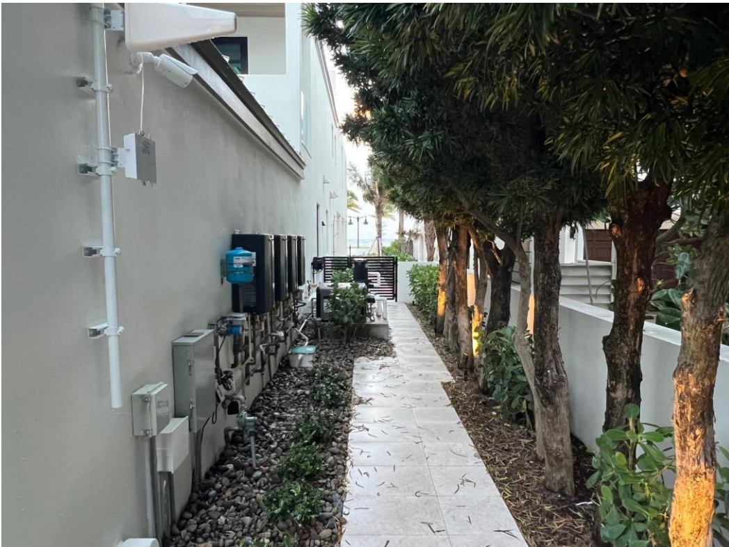
PHOTO 4: INTERIOR (SOUTH) SIDE; EAST VIEW
