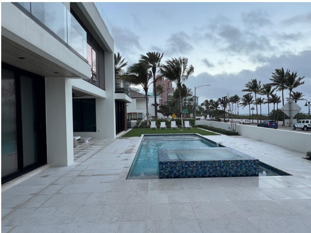
PHOTO 6: STREET (EAST) SIDE; NORTH VIEW
