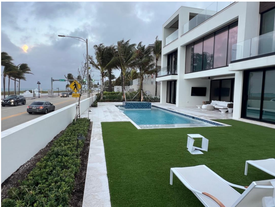
PHOTO 8: STREET (EAST) SIDE; SOUTH VIEW
