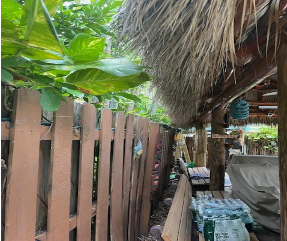
This is the East side of the chickee hut. This faces south
