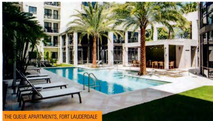
THE QUEUE APARTMENTS, FORT LAUDERDALE
