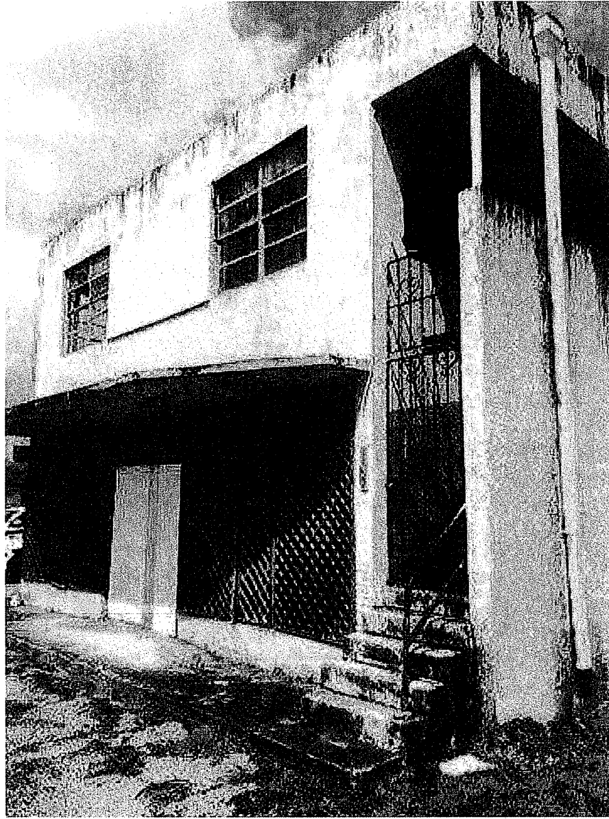
1227 Sistrunk Blvd – Existing Conditions
