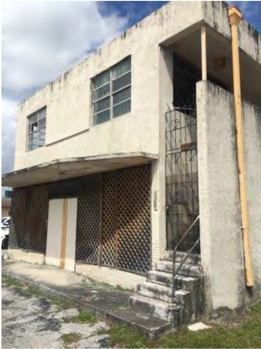
1227 Sistrunk Blvd – Existing Conditions
