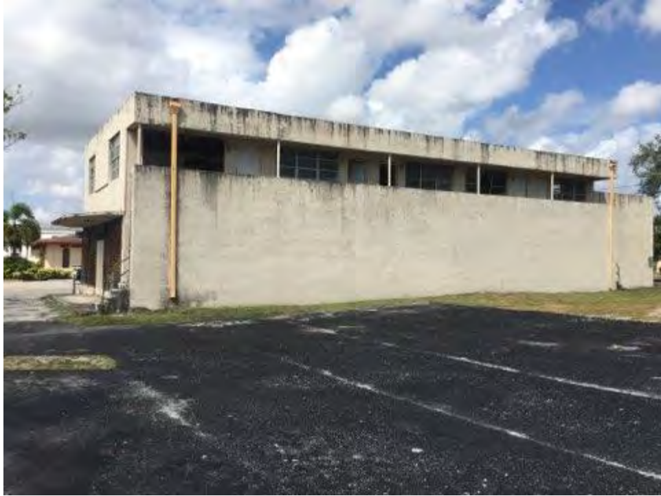
1227 Sisrunk Blvd – Existing Conditions
