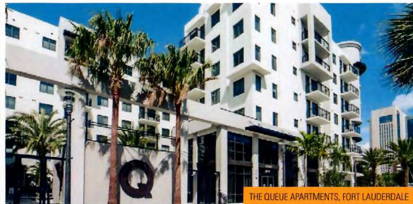
THE QUEUE APARTMENTS, FORT LAUDERDALE
