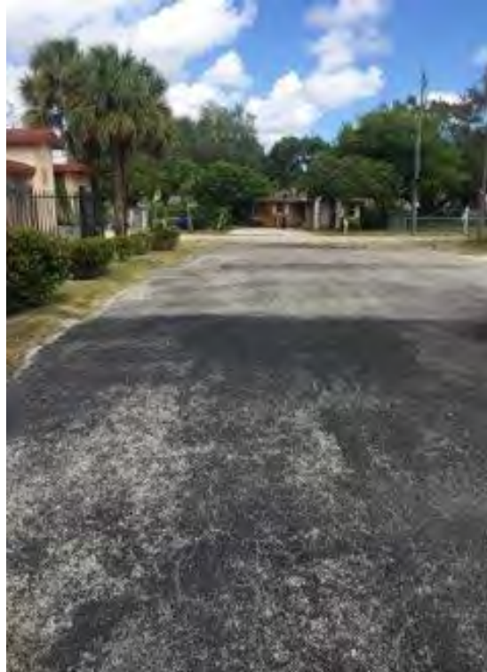
Existing Rear Parking Lot
