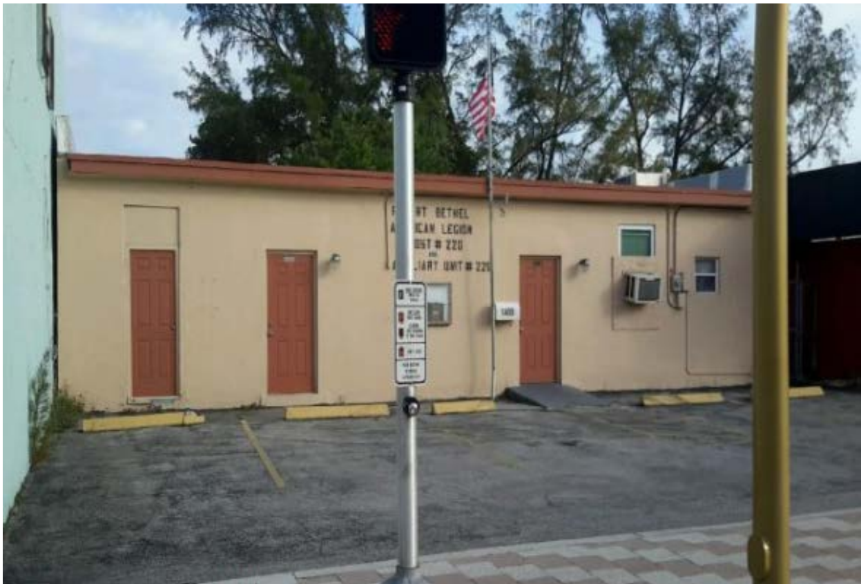
Robert Bethel American Legion Post 220 Existing Facility
