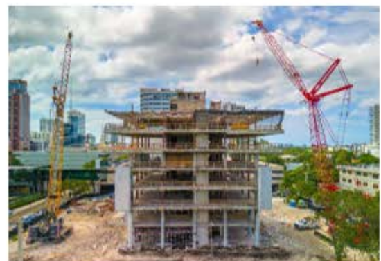
City Hall demolition site
