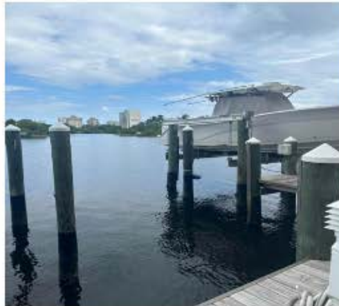
1. Subject site, showing the existing mooring pilings.
