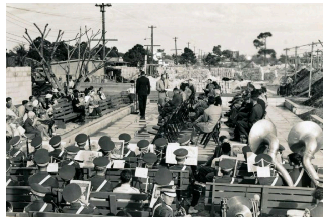
Laying corner stone at Dixie Court, December 29, 1929. Source: Fort Lauderdale Historical Society
