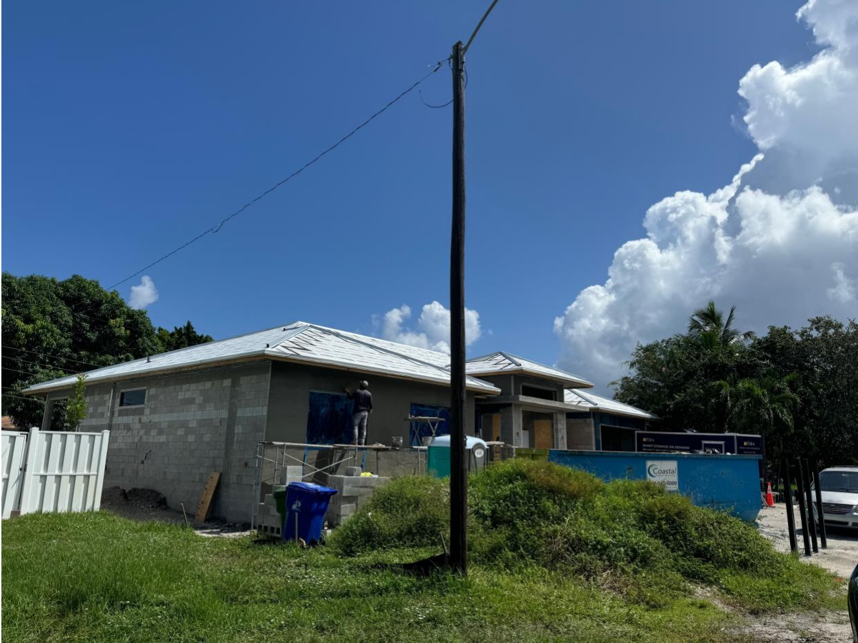
2733 NE 27 th Street West Side with Light Pole in the way of the sidewalk
