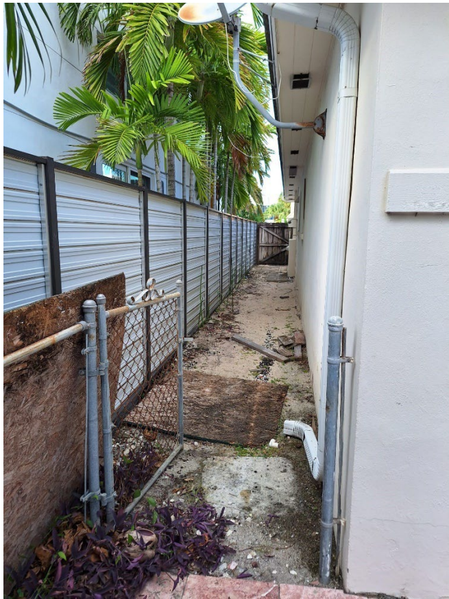
Property west view (Side) - 11.01.2023
