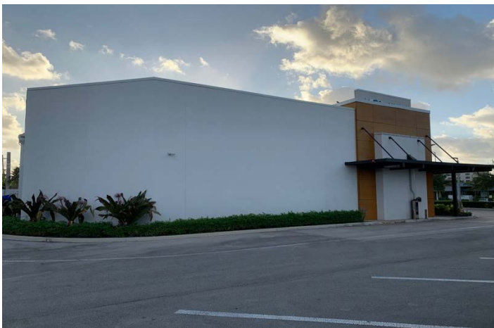
West Side of the Building
