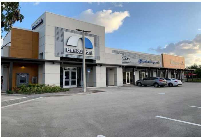
South - Front of the Building
