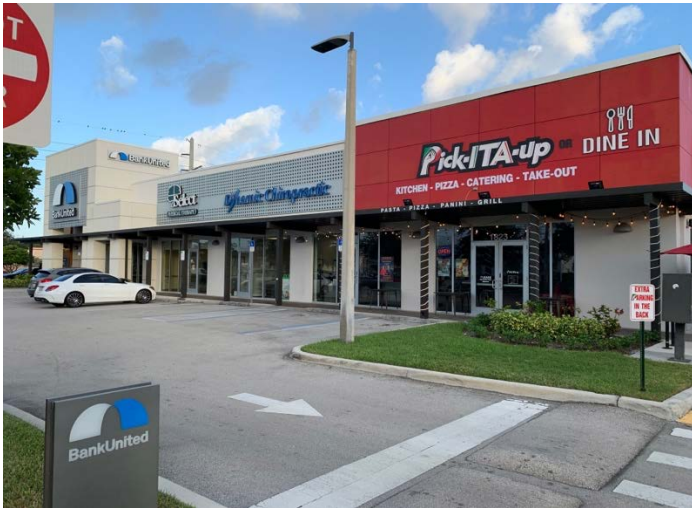
South - Front of the Building
