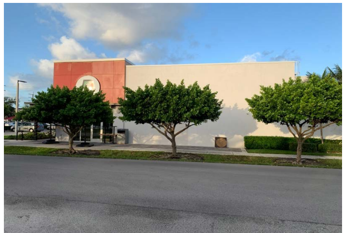
East Side of the Building
