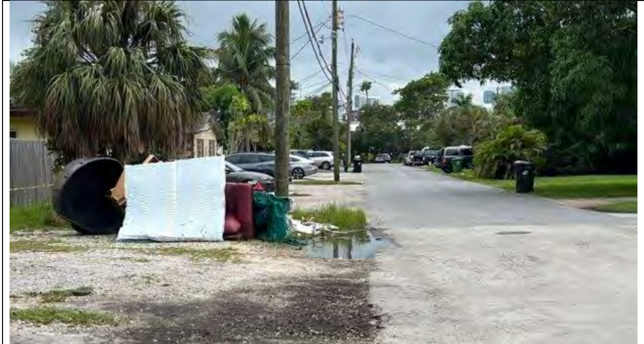
Trash and Paved Swales
