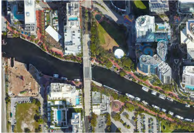
Figure 10. Andrews Street bridge showing proximity to residential high-rise buildings.
