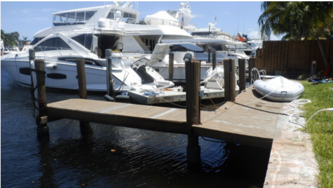
2. Northern portion of the subject site, facing south along the Middle River.
