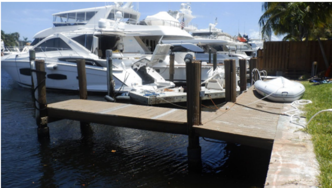
2. Northern portion of the subject site, facing south along the Middle River.
