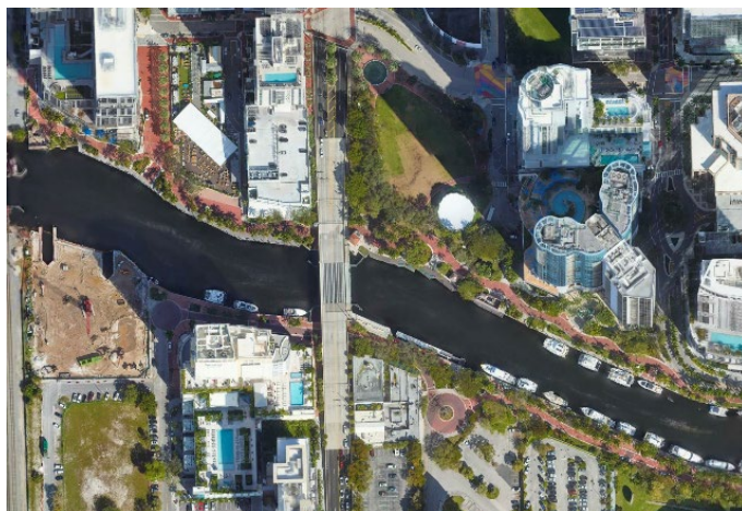
Figure XX. Andrews Street bridge showing proximity to residential high-rise buildings.
