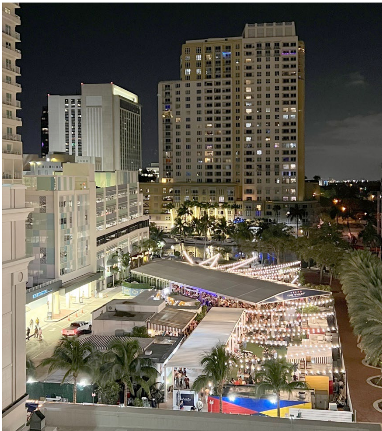
Figure XX. Aerial view of the Wharf looking south.
