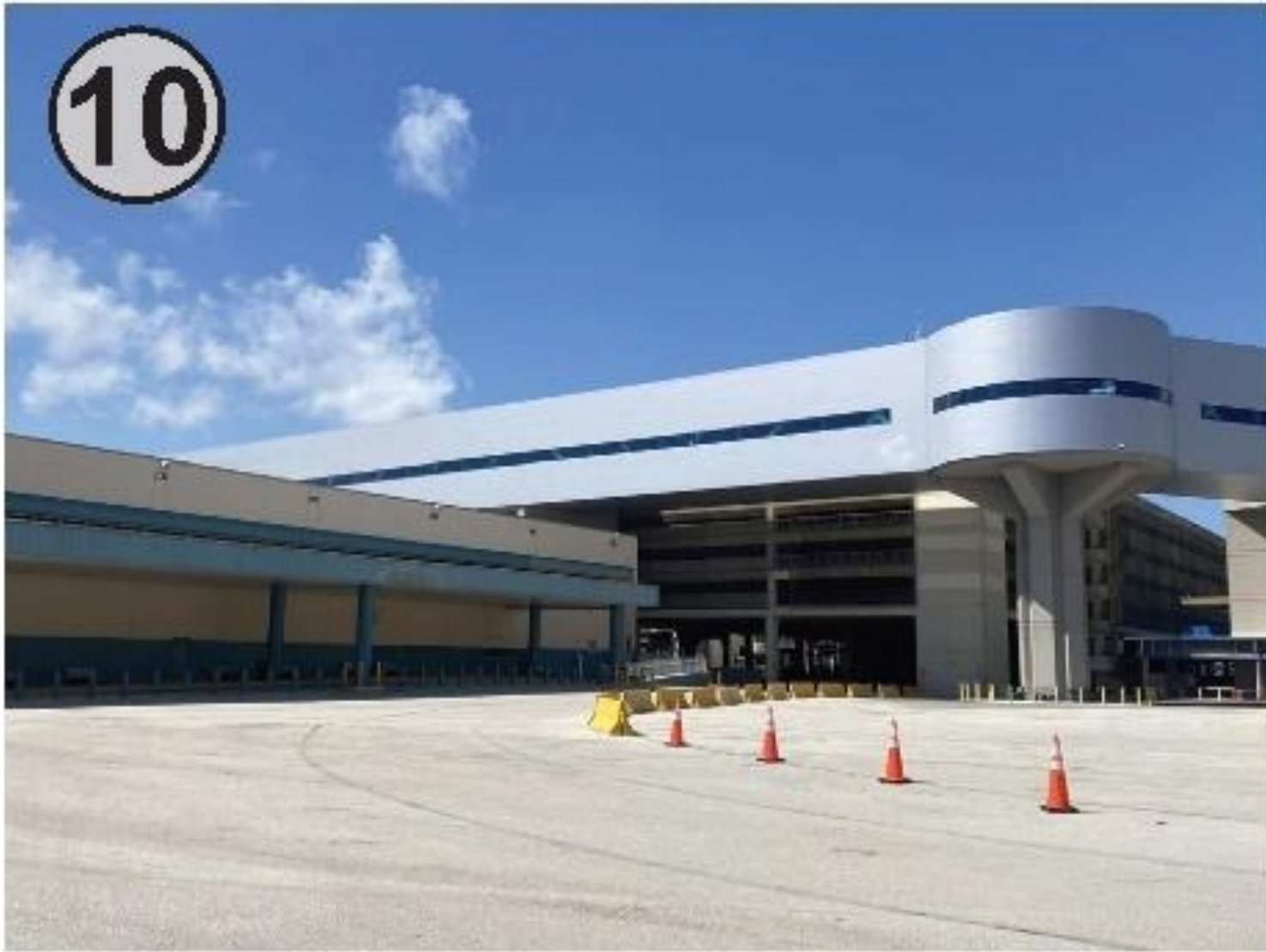
PHOTO OF TERMINAL 4 - N/E CORNER May 31, 2023
