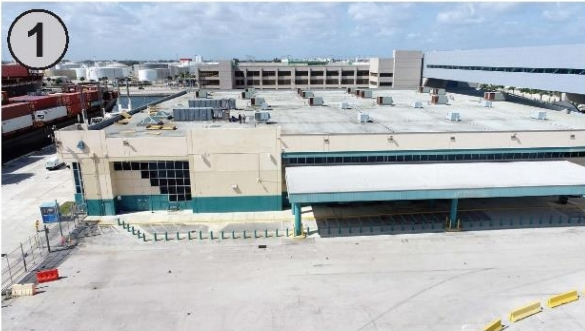
AERIAL PHOTO OF TERMINAL 4 - EAST ELEVATION May 31, 2023
