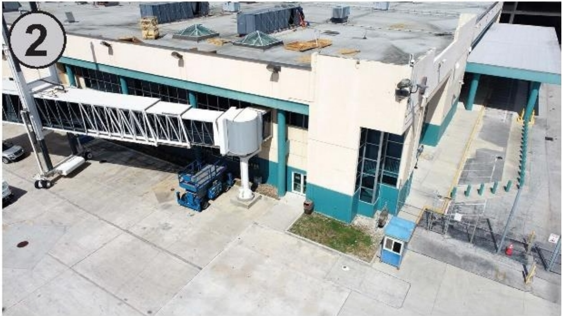
AERIAL PHOTO OF TERMINAL 4 - S/E CORNER May 31, 2023
