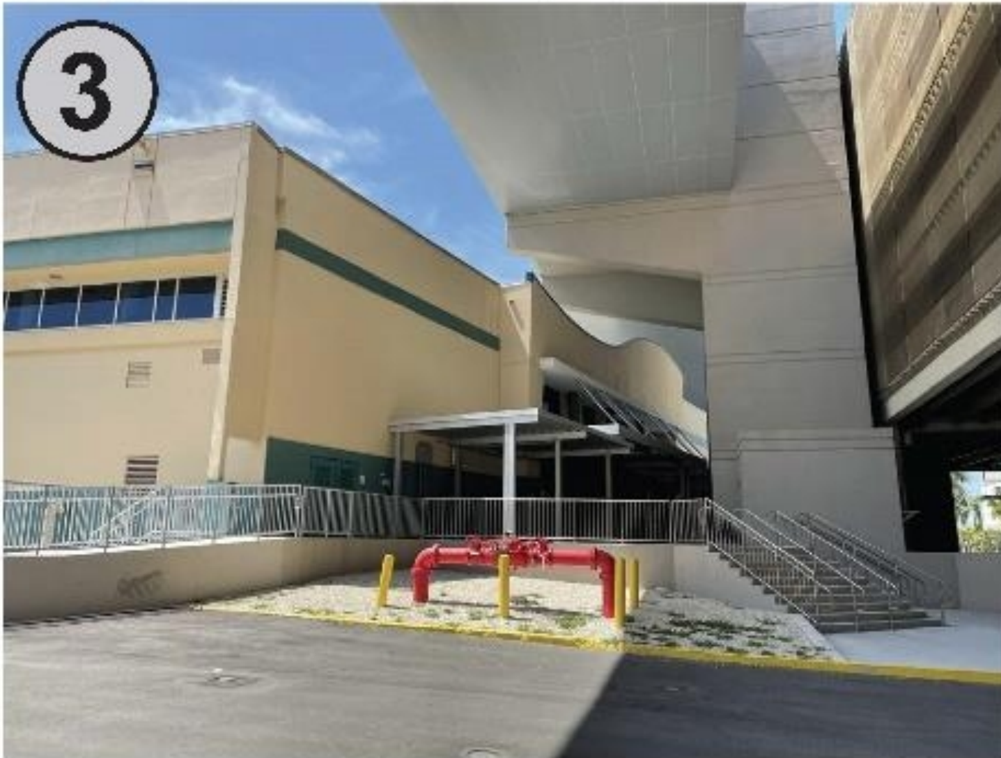
PHOTO OF TERMINAL 4 - N/E CORNER May 31, 2023
