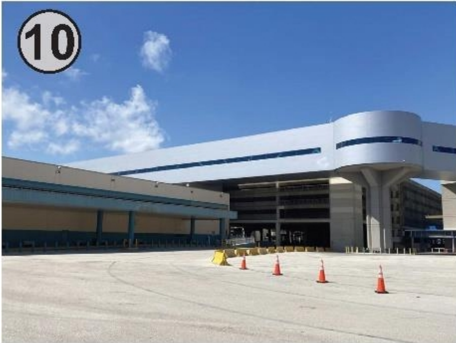
PHOTO OF TERMINAL 4 - N/E CORNER May 31, 2023
