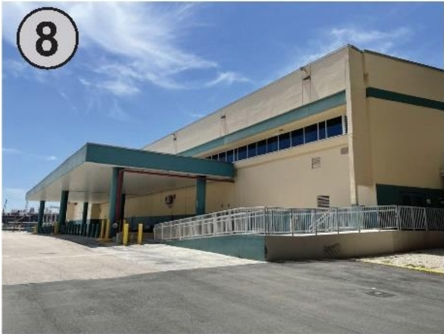
PHOTO OF TERMINAL 4 - N/E CORNER May 31, 2023
