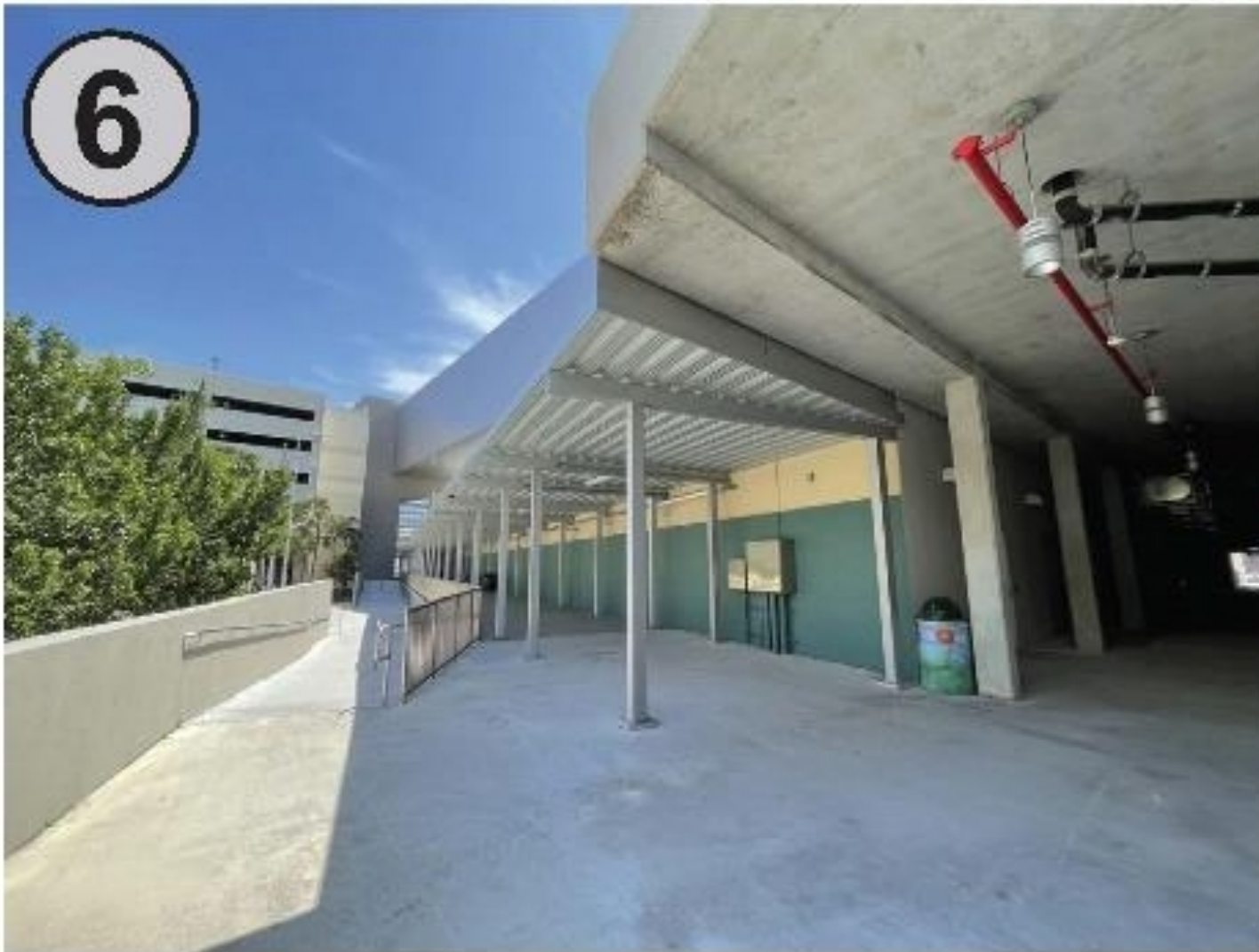
PHOTO OF TERMINAL 4 - NORTH WALKWAY May 31, 2023
