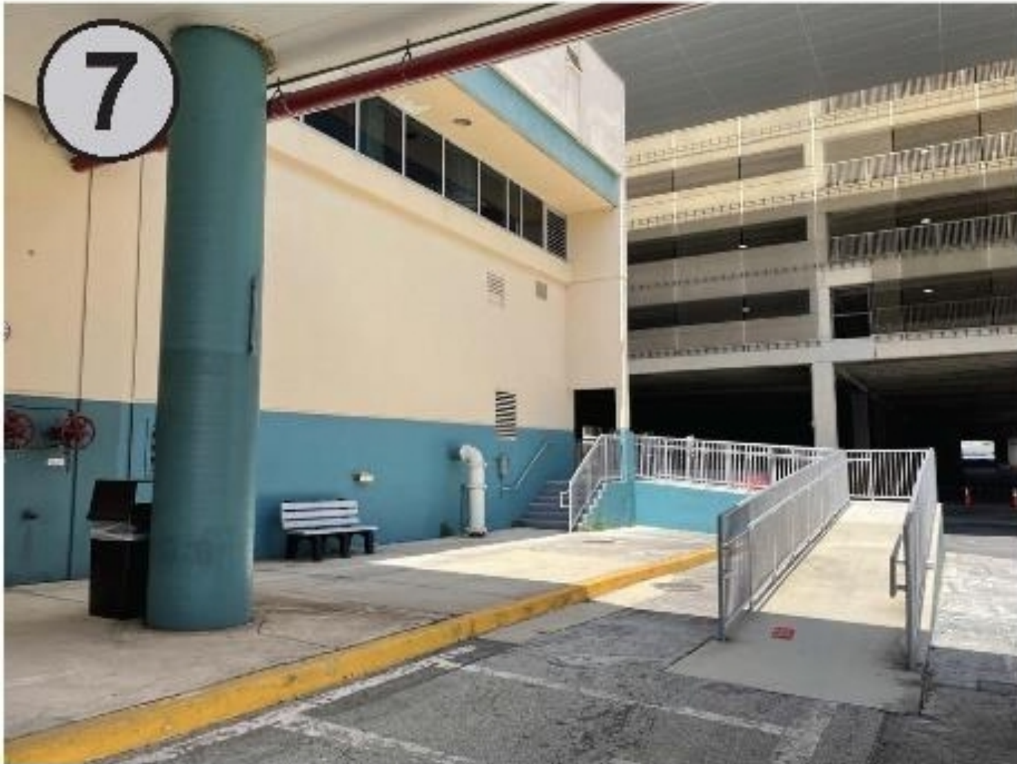
PHOTO OF TERMINAL 4 - N/E CORNER May 31, 2023
