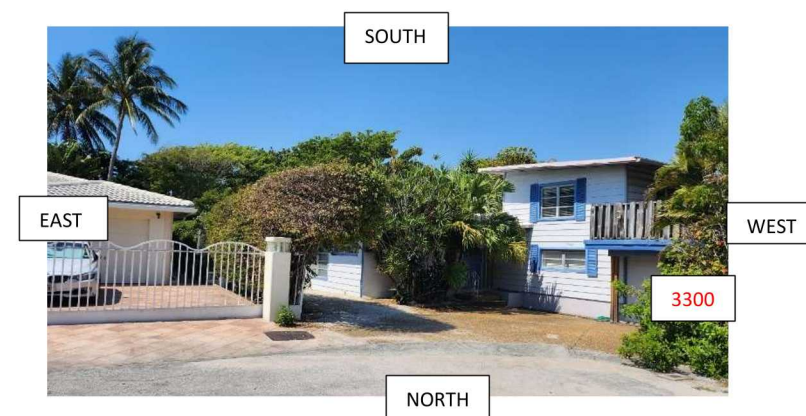
3300 NE 16 th Court (neglected property to our west) street view
