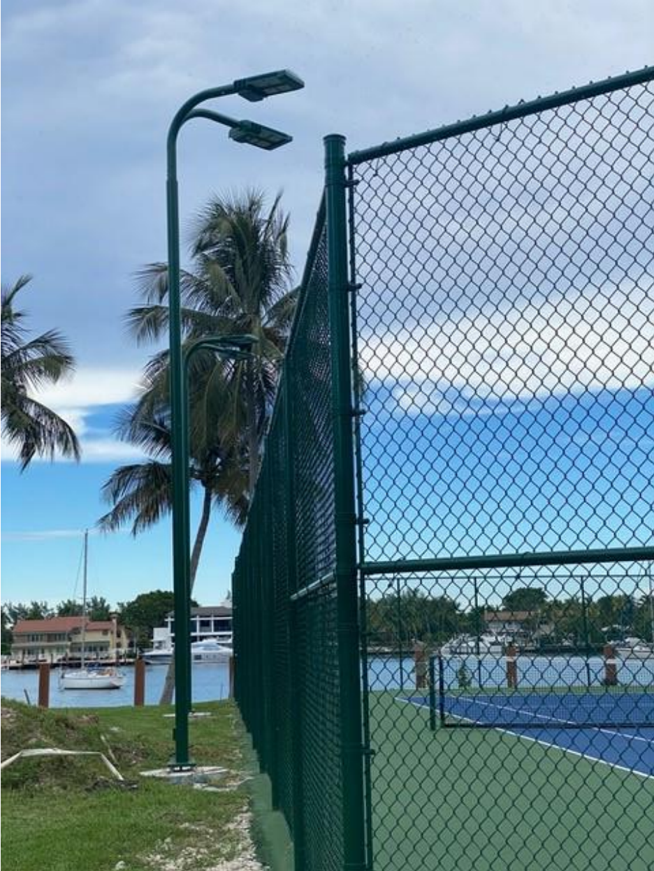
Close-up view of Tennis Court Lights
