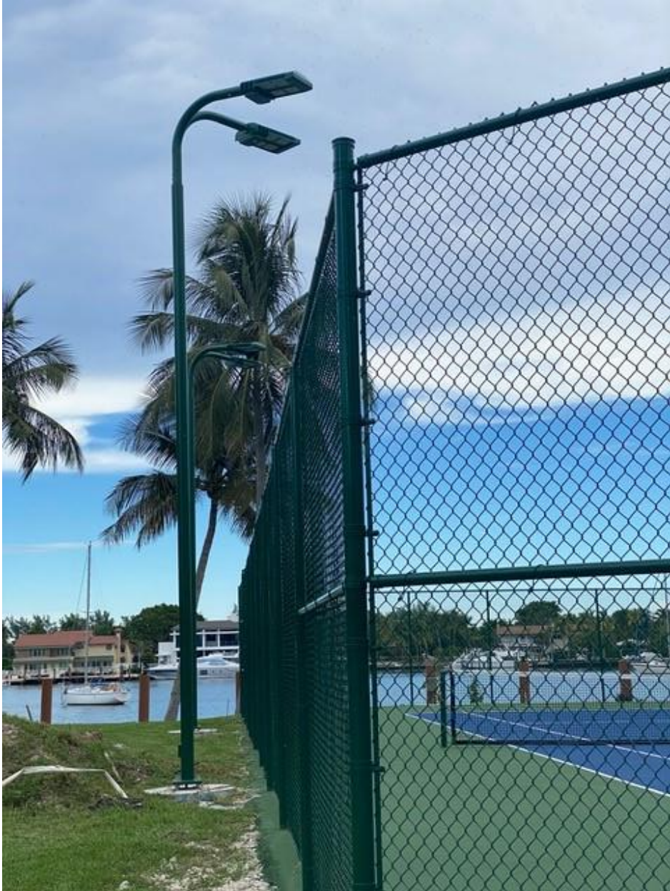
Close-up view of Tennis Court Lights
