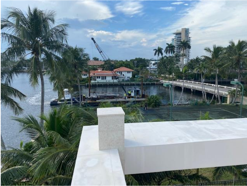
Photo of Tennis Court and Tennis Court Lighting prior to Tennis Court Replacement
