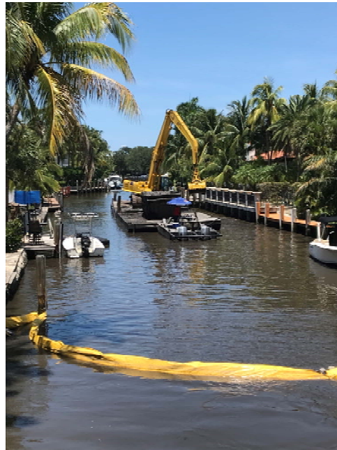
Dredging in the eastern Tarpon River
