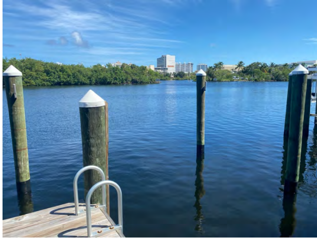
1. Subject site, showing the existing mooring pilings.
