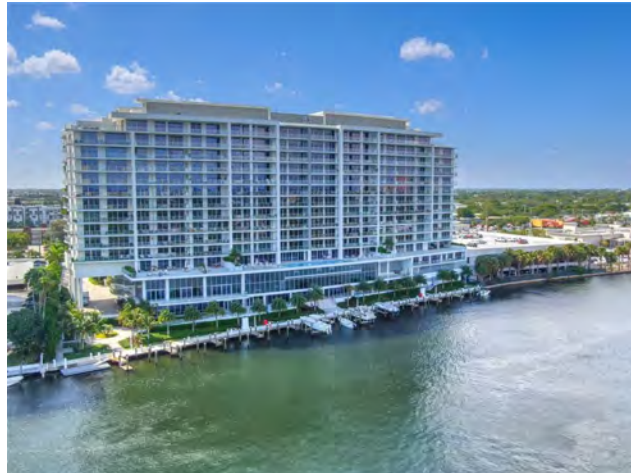
2. East portion of the subject site, facing west along the Middle River.
