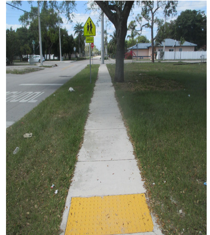
Completed Sidewalk on NW 5 th Street
