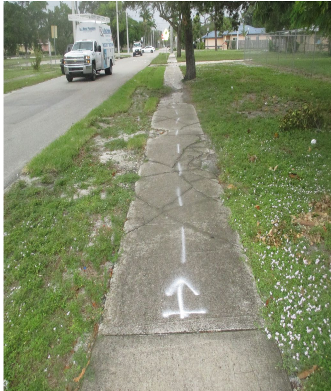
Existing Sidewalk on NW 5 th Street
