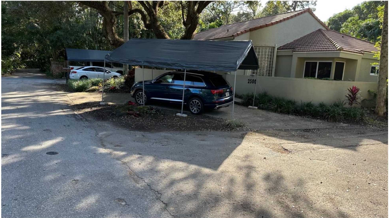
Temporary Shade Structures (Prior to removal) at 2500 SW 21 st St.
