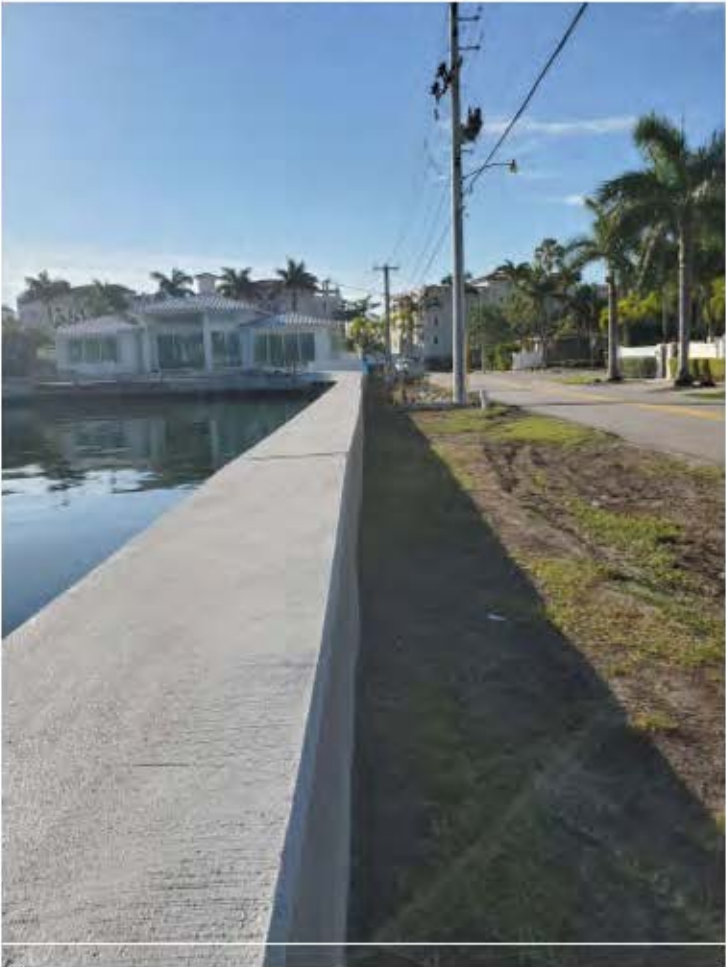
Seawall Cap from North
