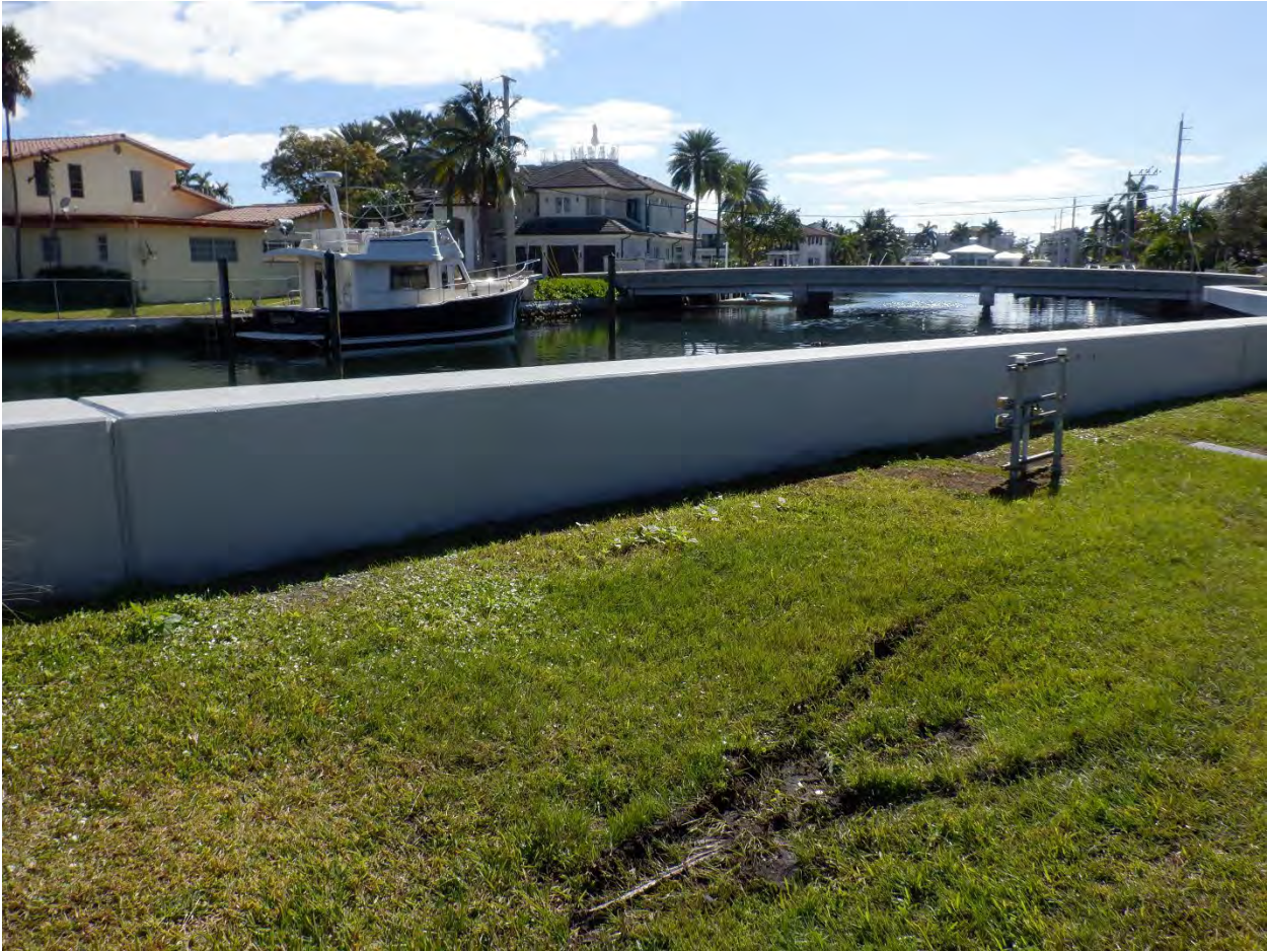
3. Central portion of the subject site, facing southeast.
