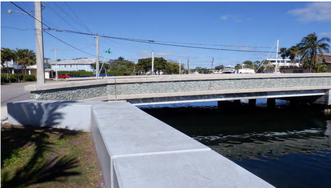
2. Southern portion of the subject site, facing north along the canal.
